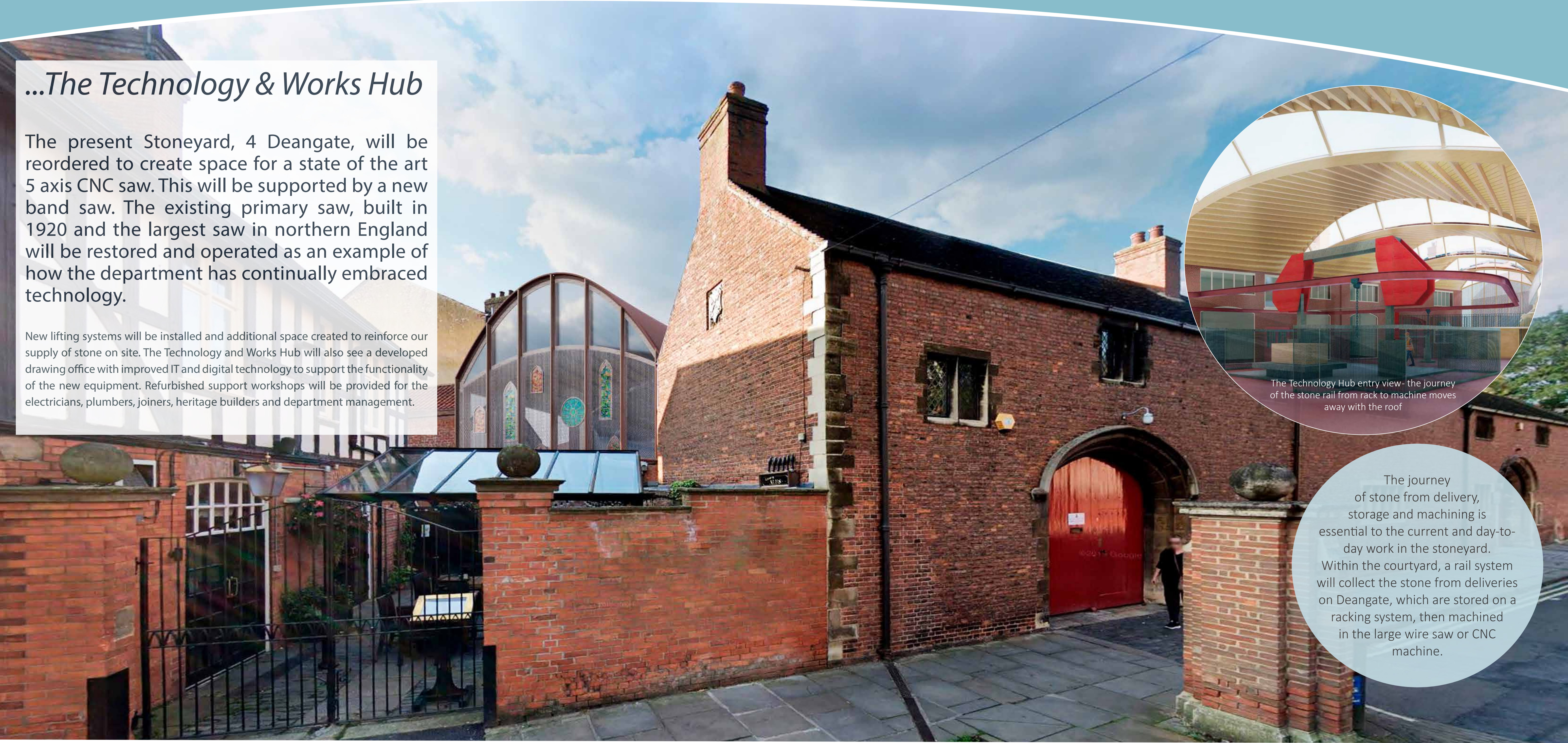
A glimpse of the new workspace will be visible on Deangate- a mesh screen provides a place for the glaziers to display work and enhances the public knowledge of the craft within
