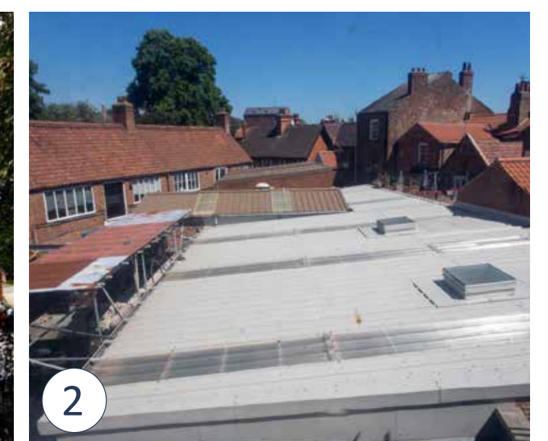
View of Courtyard Building Roof
