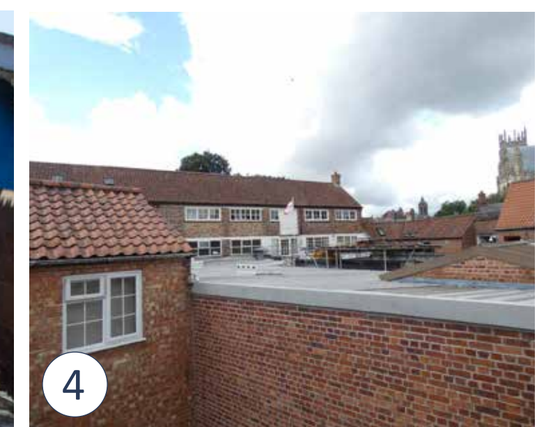
View of wall to rear of properties on Goodramgate
