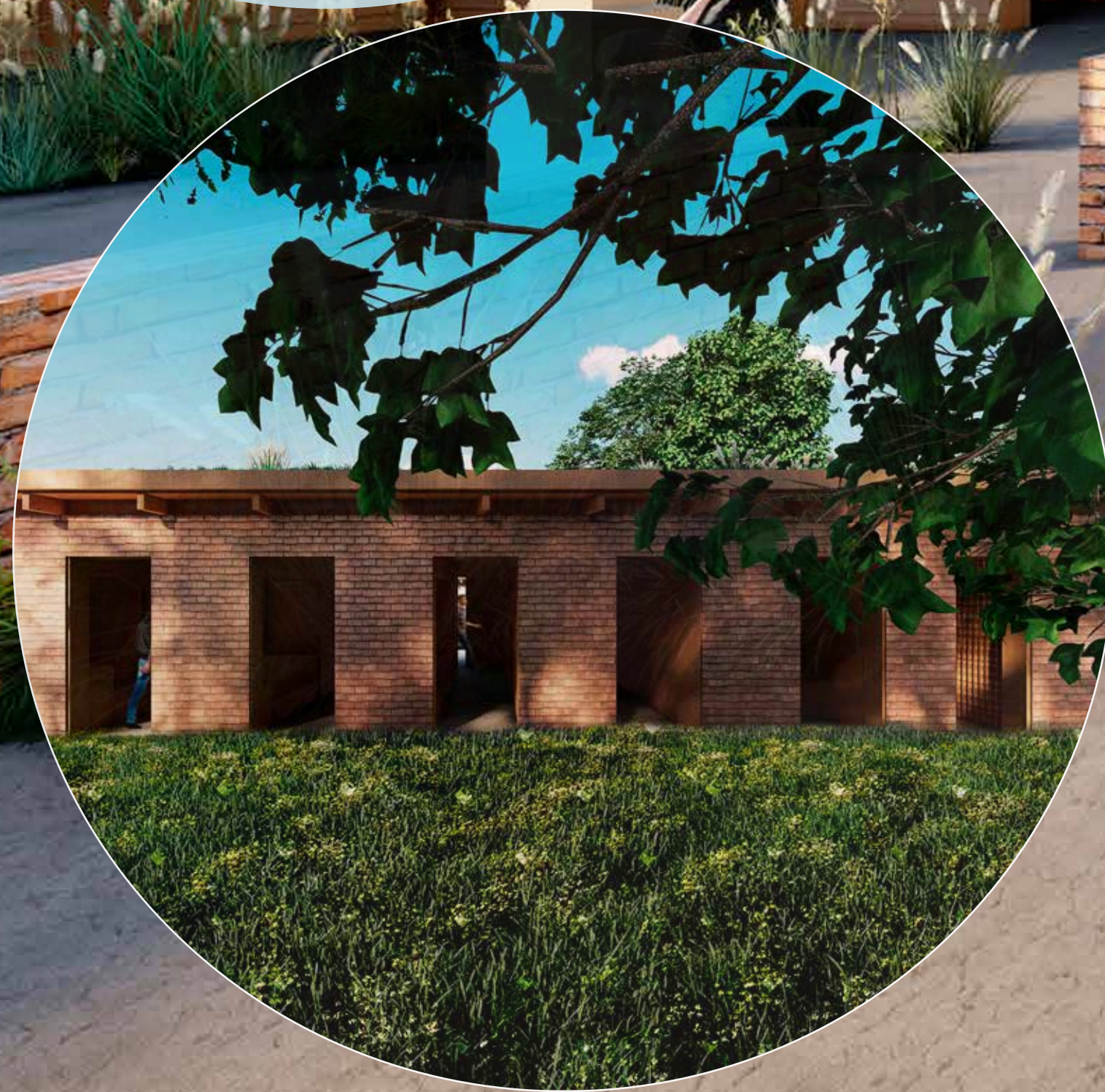
Outside of the courtyard, the walls are clad in reclaimed tiles from the existing roof and similar to match.
