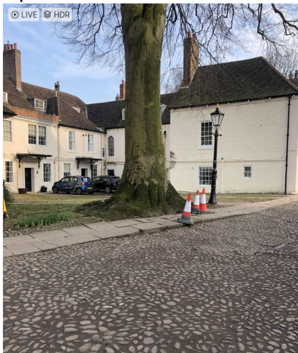
Plate 1. Area of paving lifted by tree roots.
