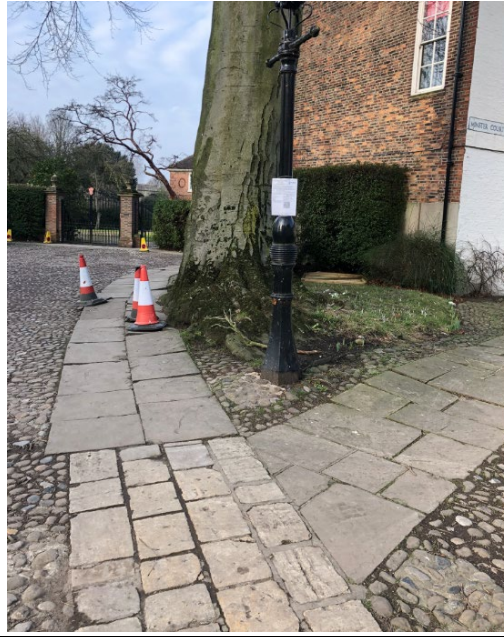
Plate 4. Extent of flags to be replaced
