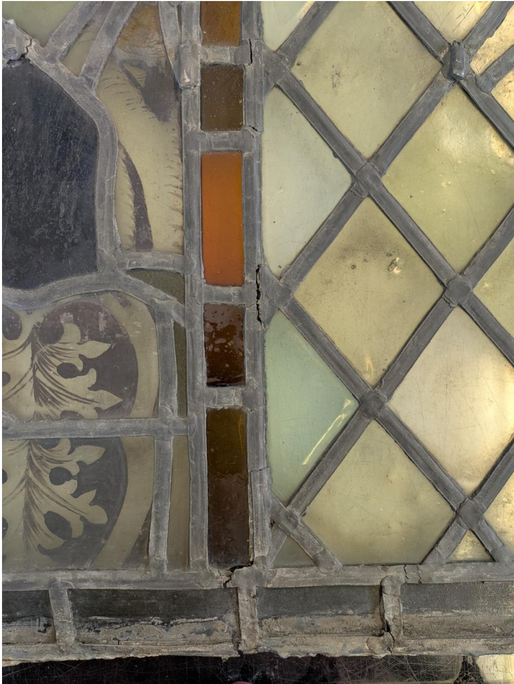
Fig.4: Failed solder joints, s20
