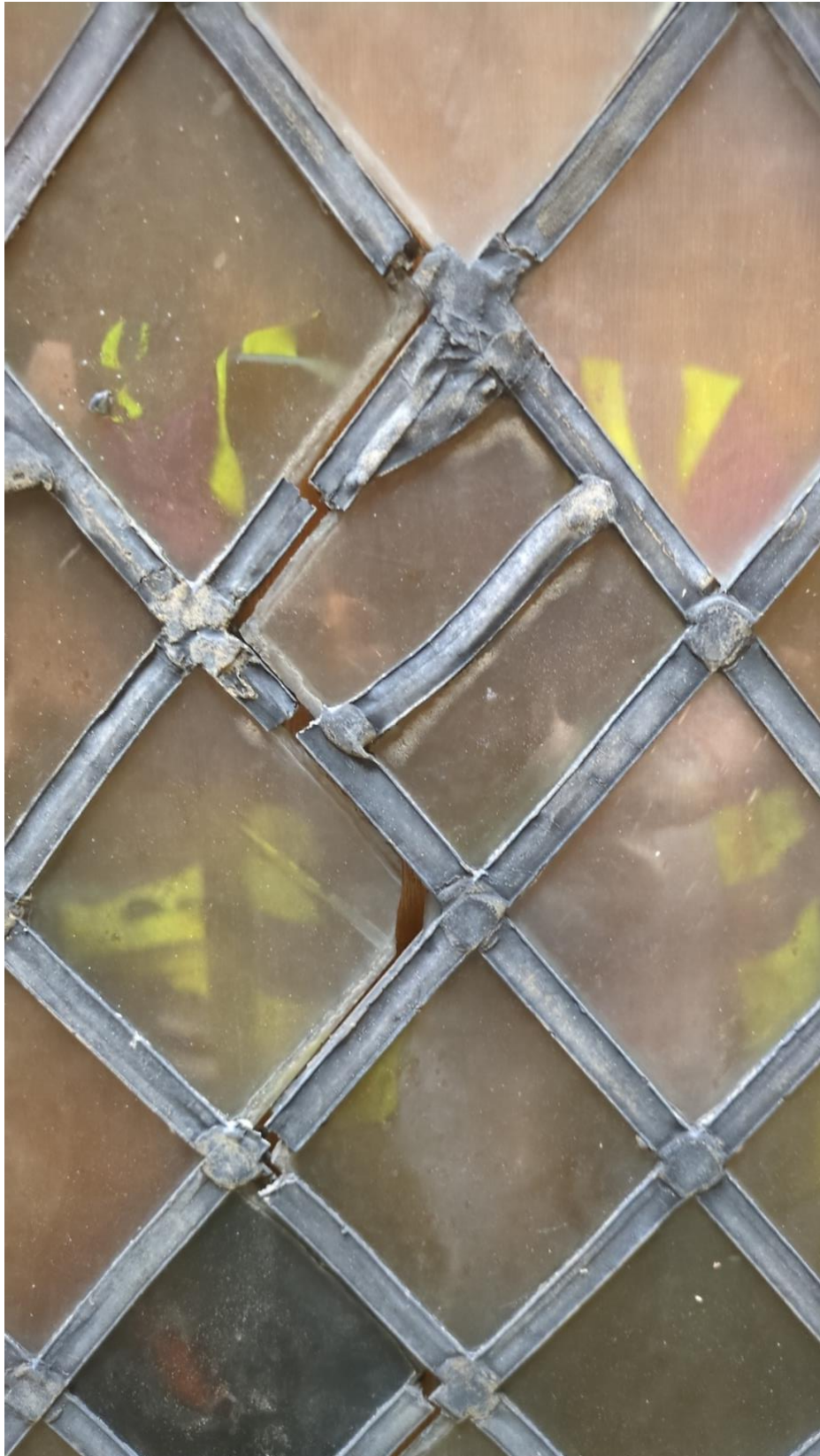
Fig. 3: Broken Solder Joints, s20
