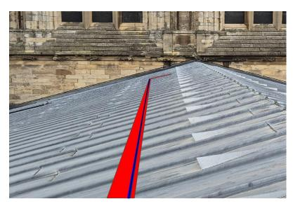
The Starlink dish will require a single RJ45 data cable, which will be routed along the existing 100 mm cable tray beneath the photovoltaic (PV) installation
