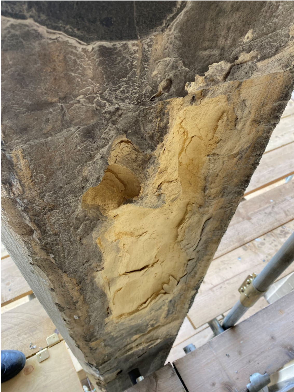
Preferential decay of softer units in the primary skeleton structure.
