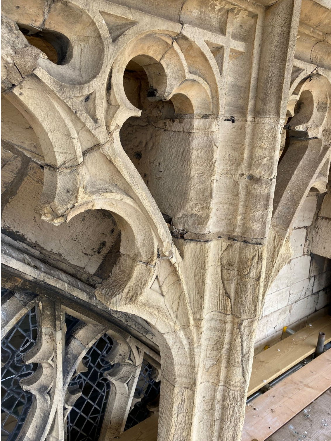
Cracked and spalling stones – note the enlarged bed joints which conceal rusting iron.
