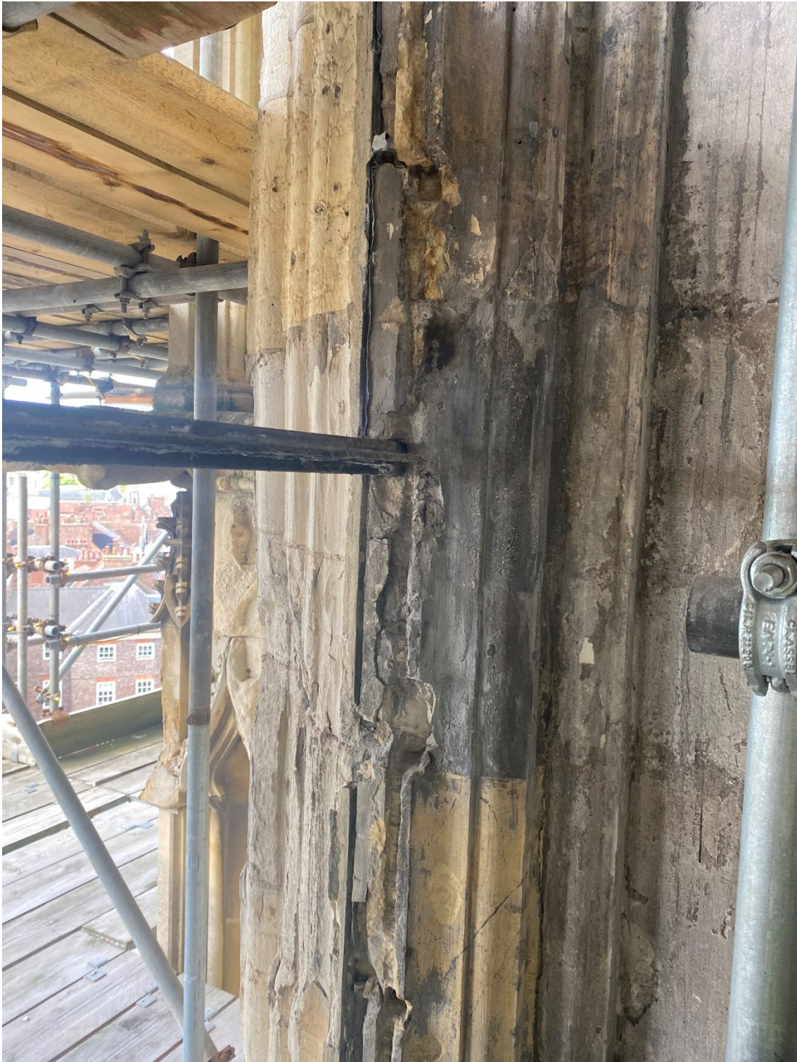
Damage to the stonework along the glass line and the very extensive cementitious 'repairs.'
