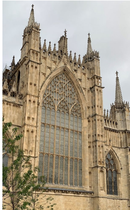
Left: Photograph showing completed pinnacle repairs incorporating a mixture of Cadeby and Highmoor stones. Right: Photograph showing precedent use of Lepine
