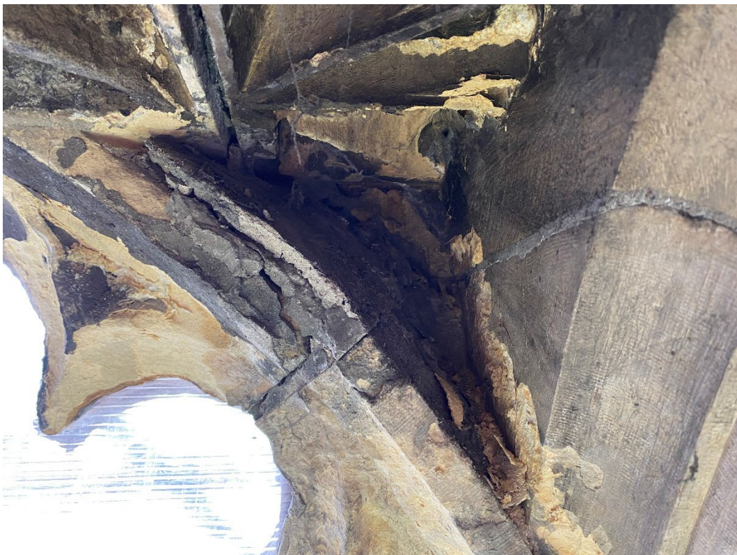
Fractured, spalling and friable stonework internally, again creating a safety issue by presence of loose and detaching fragments.
