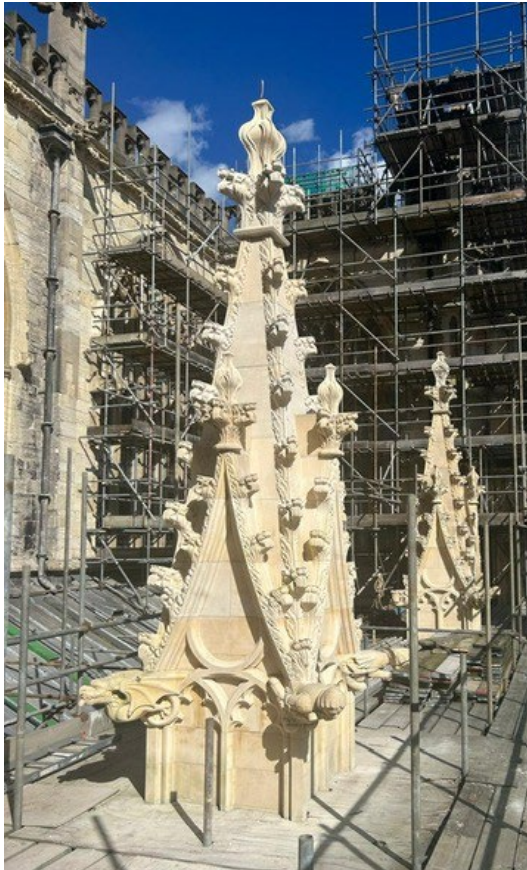
Left: Photograph showing completed pinnacle repairs incorporating a mixture of Cadeby and Highmoor stones. Right: Photograph showing precedent use of Lepine
