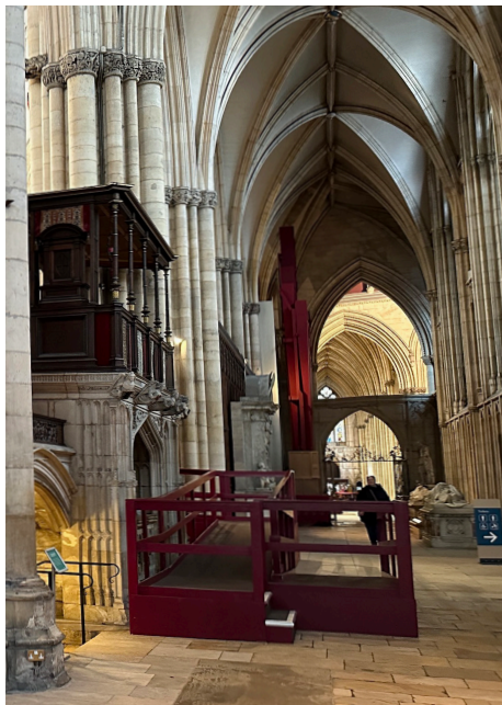
Temporary ramp installed between Quire and Upper Quire
