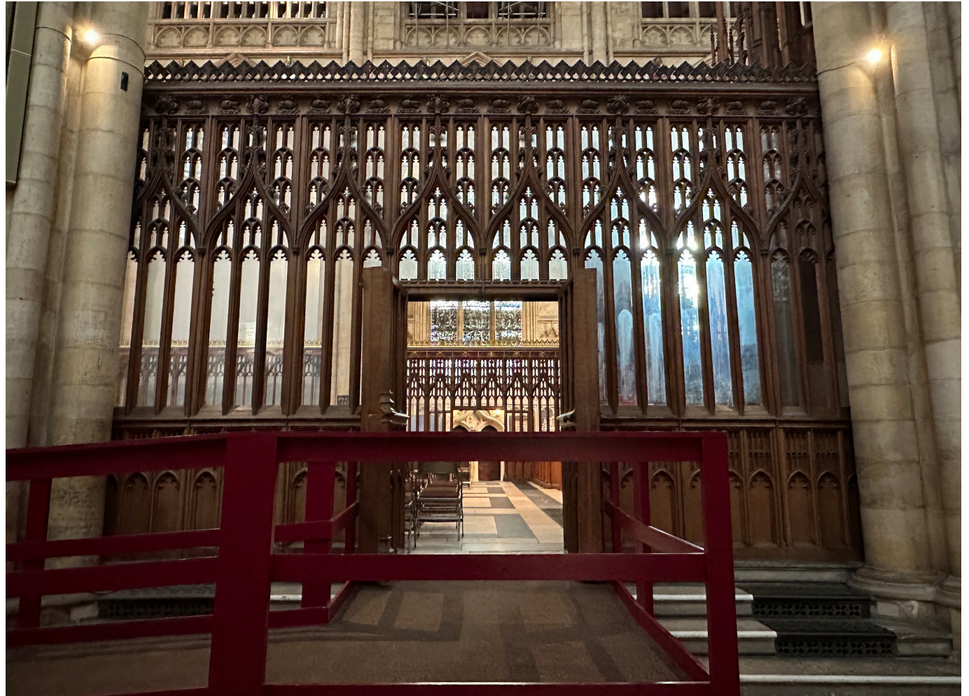
North Quire Aisle ramped entrance to the Upper Quire
