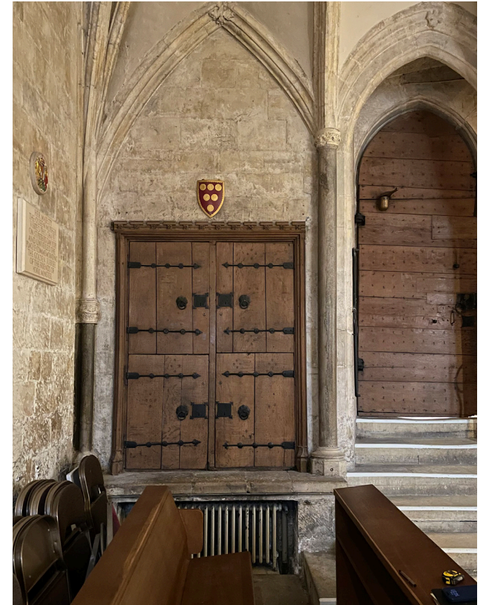
N Elevation, historic timber cupboards, used for storage
